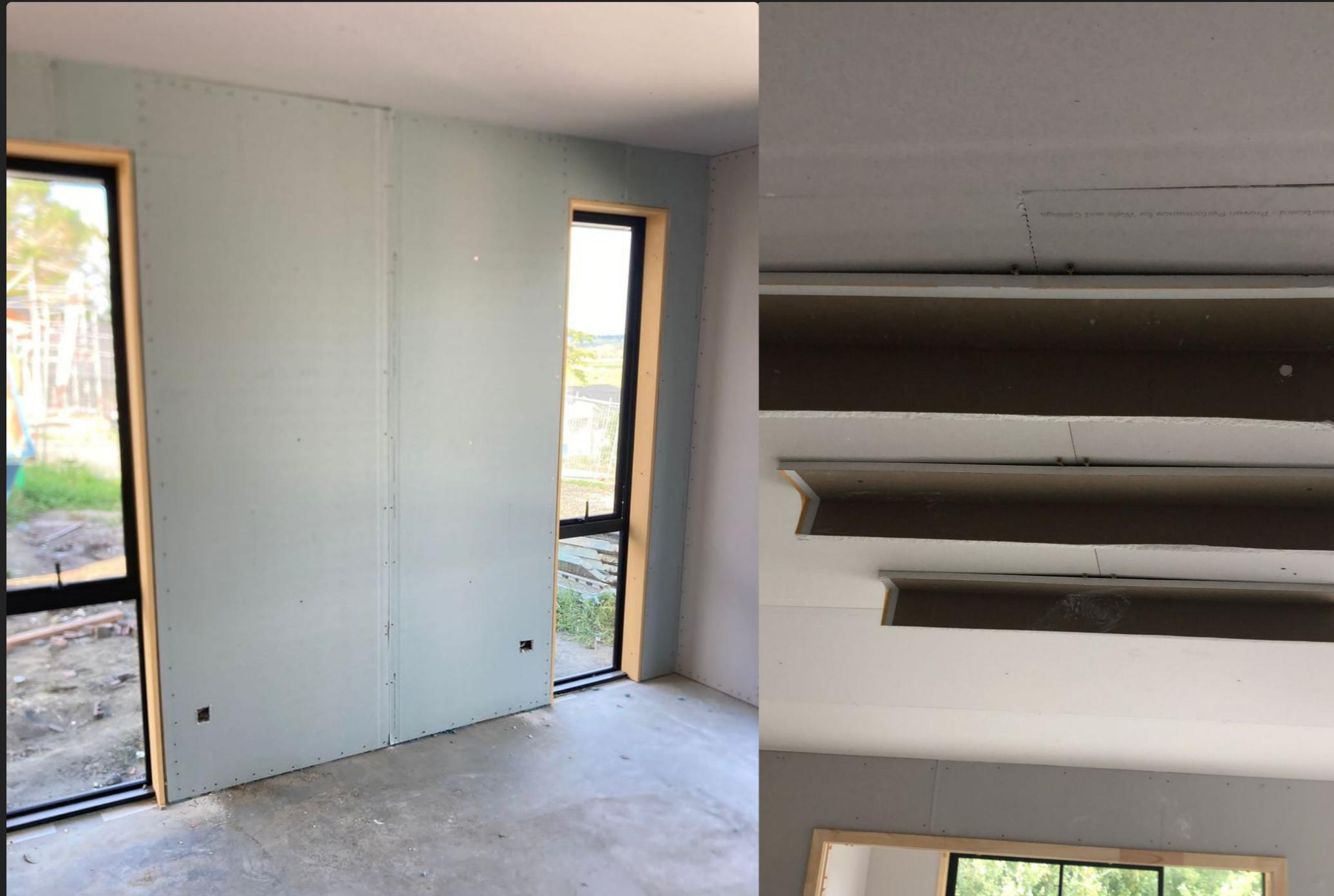
For both residential and commercial projects, our GIB fixers ensure walls are lined horizontally whenever possible, following the GIB Guide to minimize joints and plastering, resulting in a high-quality finish.
