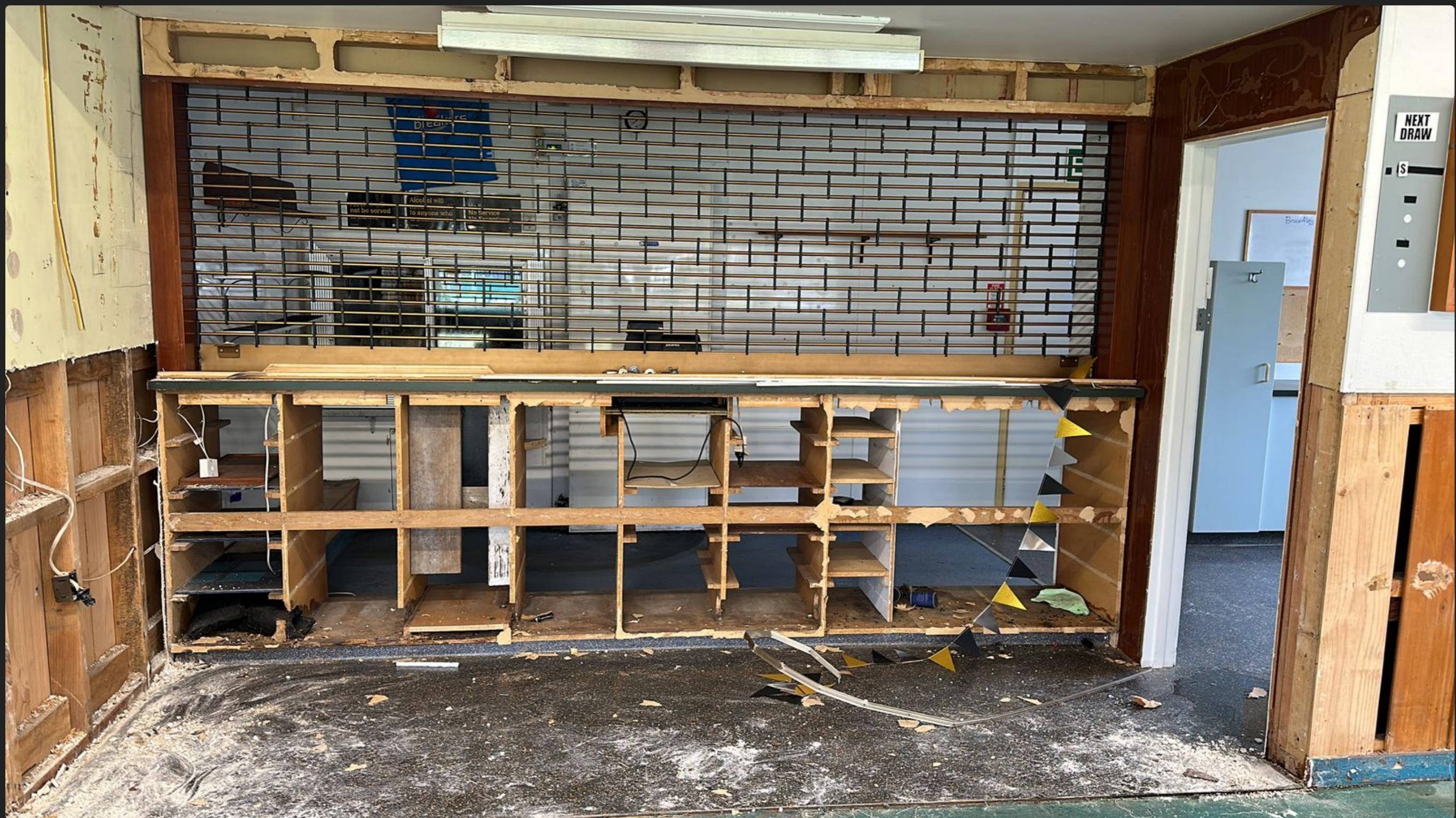
“Unfortunately, Mairangi Bowling Club was also affected by flooding. But no worries! We carried out a full renovation of the bar, kitchen, and function area including a new layout of bar, new doors, frames, and hardware, new huge sliding doors, a new kitchen, a new storage room, new flooring (vinyl, carpet, and polished floors), roofer crew, and managed the Chem Dry crew, among other tasks.”
